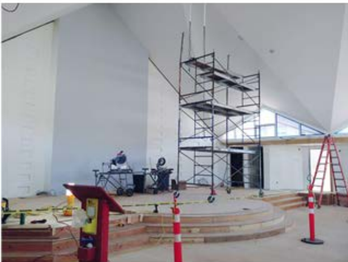
Chancel area of the sanctuary.
