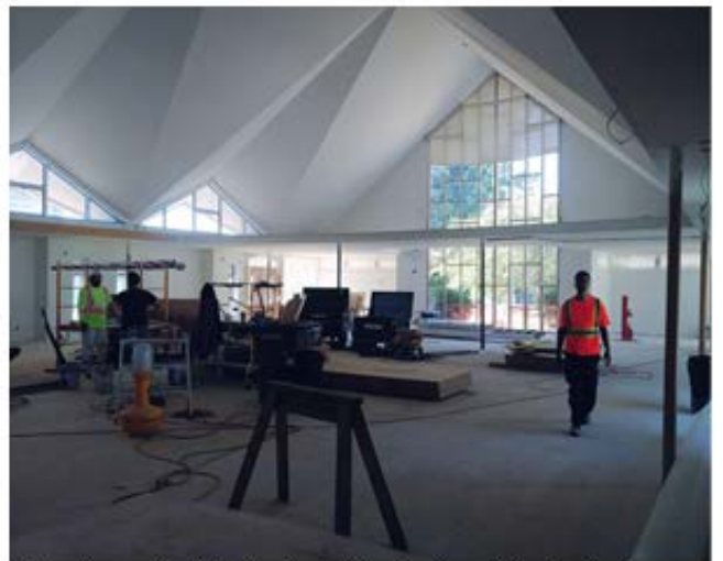
Sanctuary, looking to where the Narthex is beginning to take shape.
