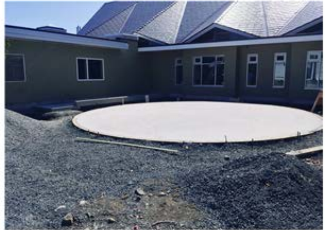
Concrete Pad has been poured for the new labyrinth.
